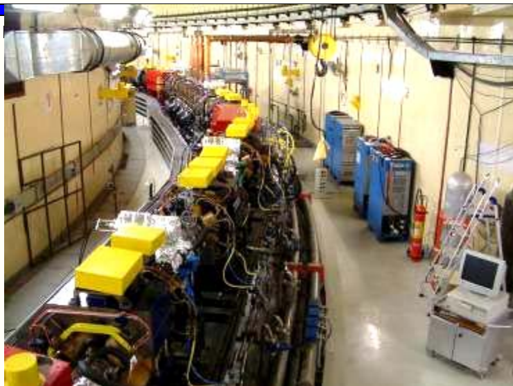
Indus-2 Ring in the Tunnel
